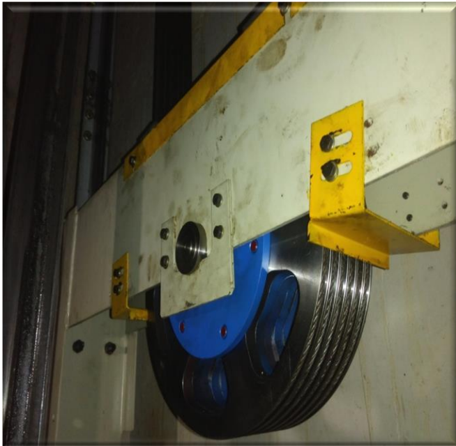
Weight side "divided independent rope pulley" installation example
